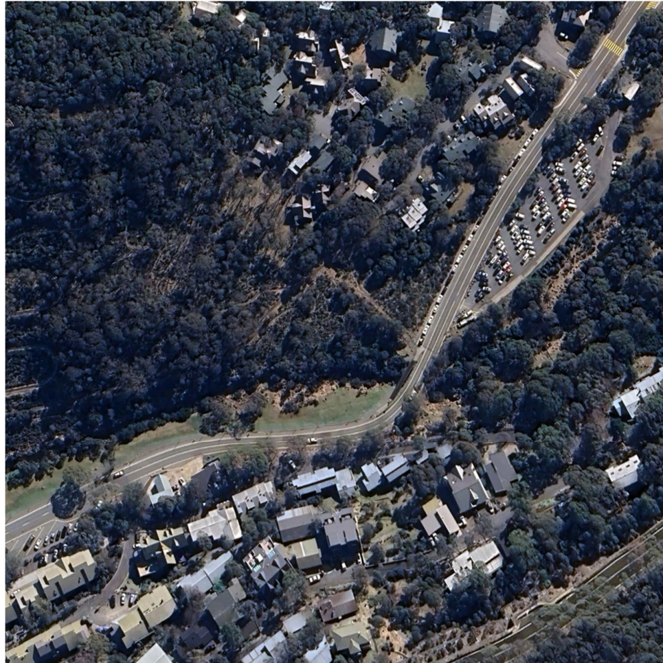
Figure 13: Existing carparking located to the north of the site.
