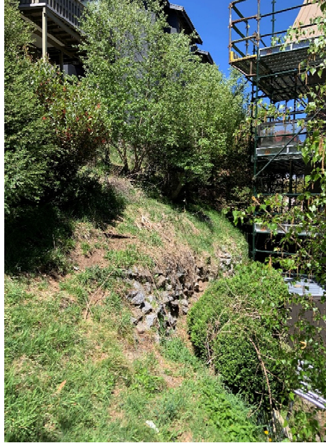
Figure 9: Rear retaining wall at the Ullr rear courtyard, Image taken from the boundary of the proposed site
